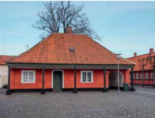
When the garrison vacated Hammershus in 1743, people started to use the walls as an ersatz quarry, and thousands of bricks were pilfered before the castle was placed under a preservation order in 1822. Hovedvagten, the main guardhouse, in Rønne, which is painted red, was built in 1744 for military purposes. It is without doubt one of the buildings constructed using bricks from Hammerhus, which makes it a prime example of brick’s sustainability and recycling potential.
