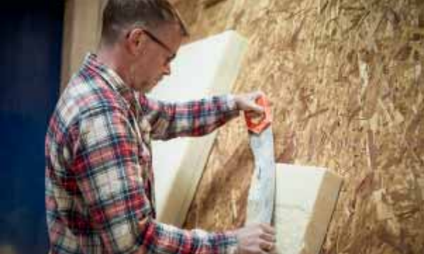
1. Cutting the polyurethane casting mould.
