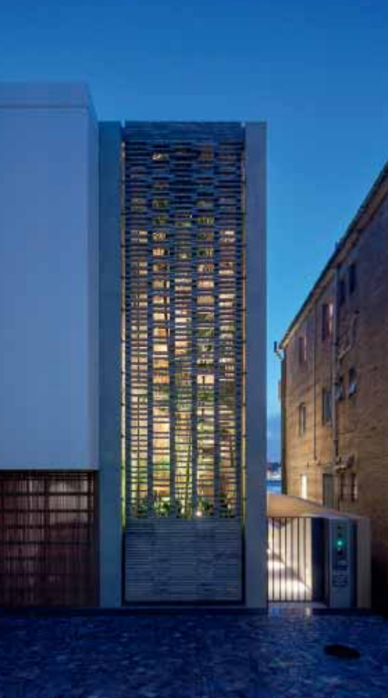
The building’s character changes at night, when the decorative screens resemble a lantern in the dark.
