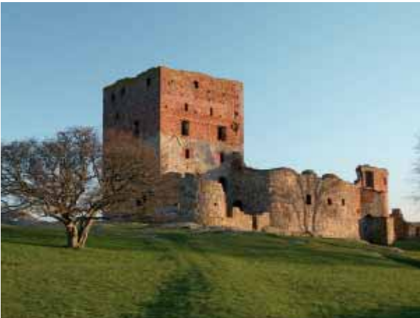
Work on Hammershus on the Danish island of Bornholm started in the 13th century. The bricks are from various periods, but the majority were produced in the 16th and 17th centuries. Stamps show that many of them came from Lübeck, which ruled Bornholm for about 100 years. The ones without stamps were most probably made on the island.
