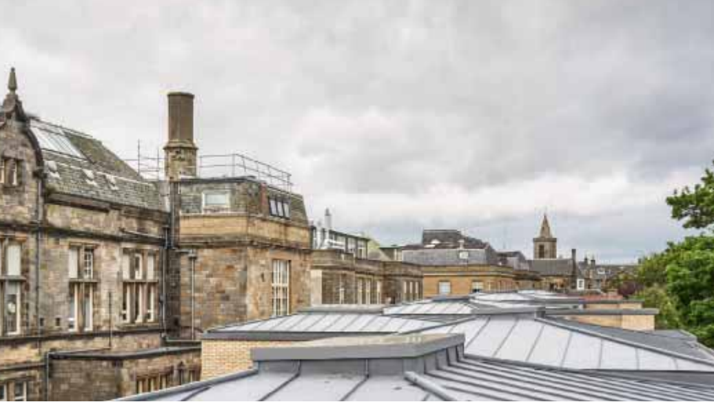
The new building is one storey lower than the neighbouring Bute Building, built in 1897, which is the oldest medical faculty in Scotland.
