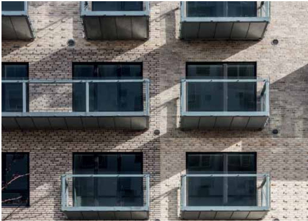
The same brick is used throughout, but the look varies greatly due to different bonds and joint colours, and because in some places the headers protrude from the façade.
