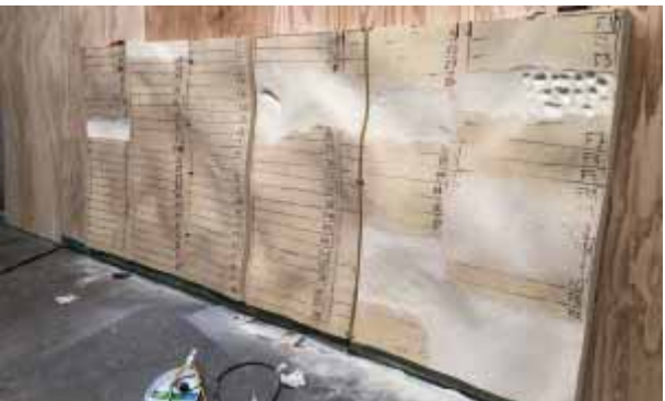
12. The moulds are ready to be copied in negative, for use in casting the concrete panels.
