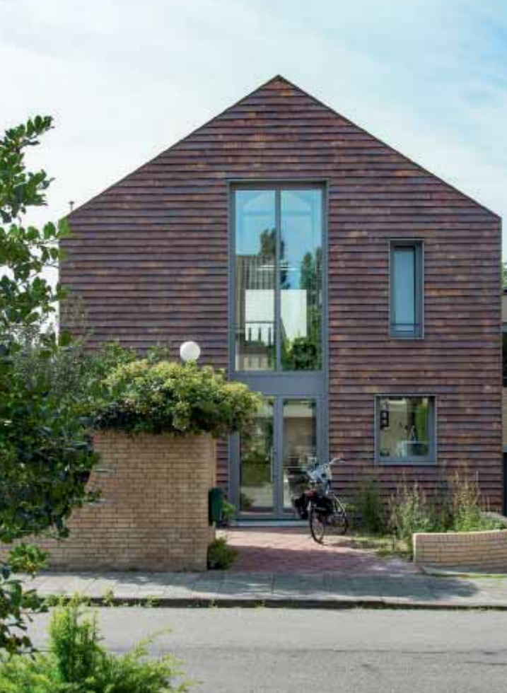
A protruding glass panel on the front façade was removed and replaced with a slightly retracted main glass panel.
