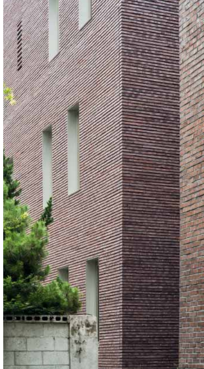
For the façades, the architects and clients chose a handmade, red-brown brick that stands out by virtue of its format, structure and colouring.
