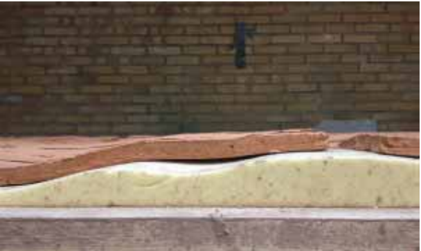
9. The fired bricks are not fully aligned with the moulds, which must be adjusted later.
