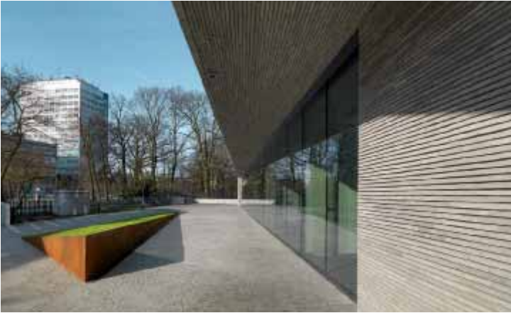
To the south, the ground floor is retracted. Like the façade, the underside of the cantilevered first floor is clad in Kolumba. Photo: Wojciech Krynski.
