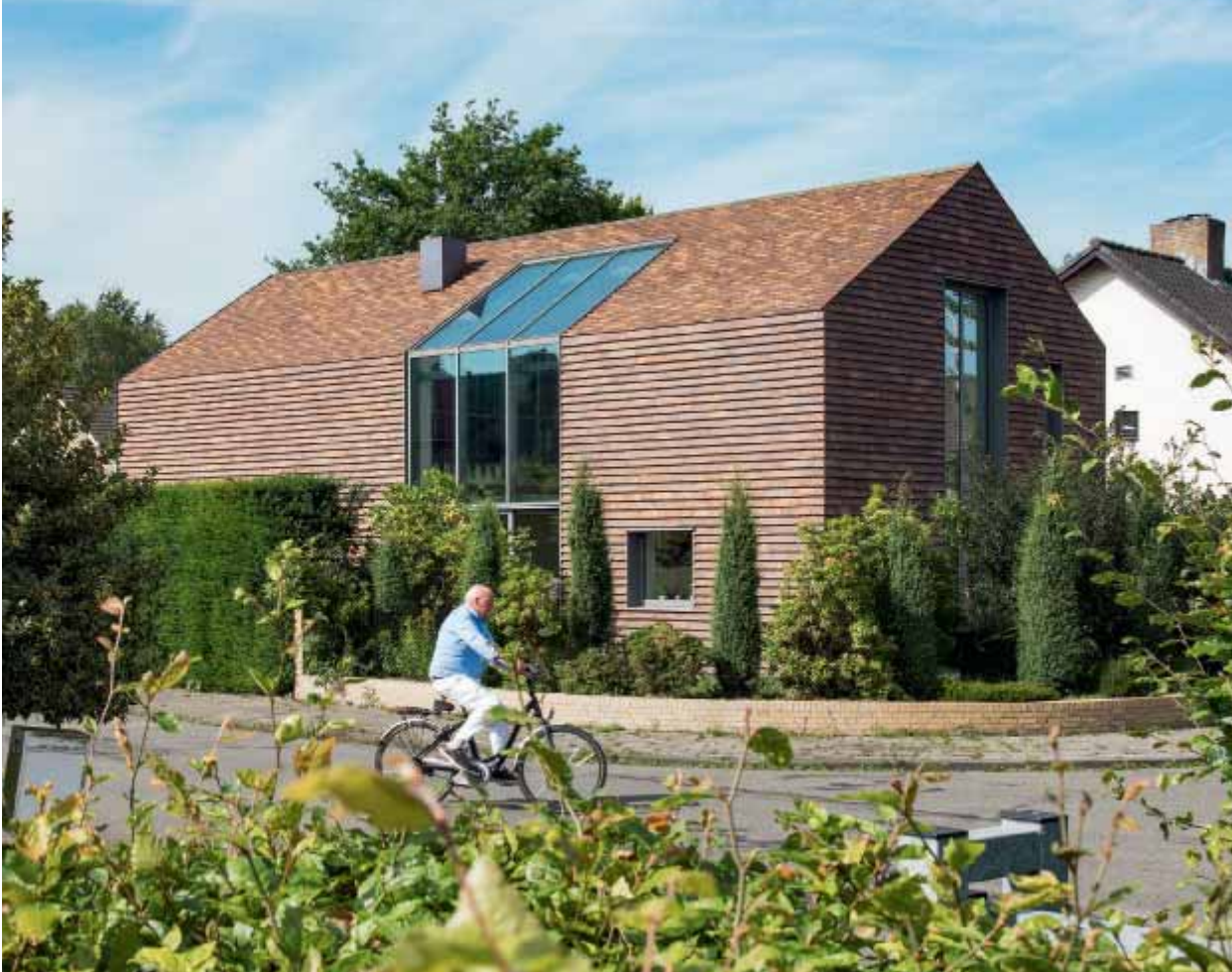
The architect wanted minimal perforation in the brick cladding. The façade to the east features a single large glass section that extends onto the roof.
