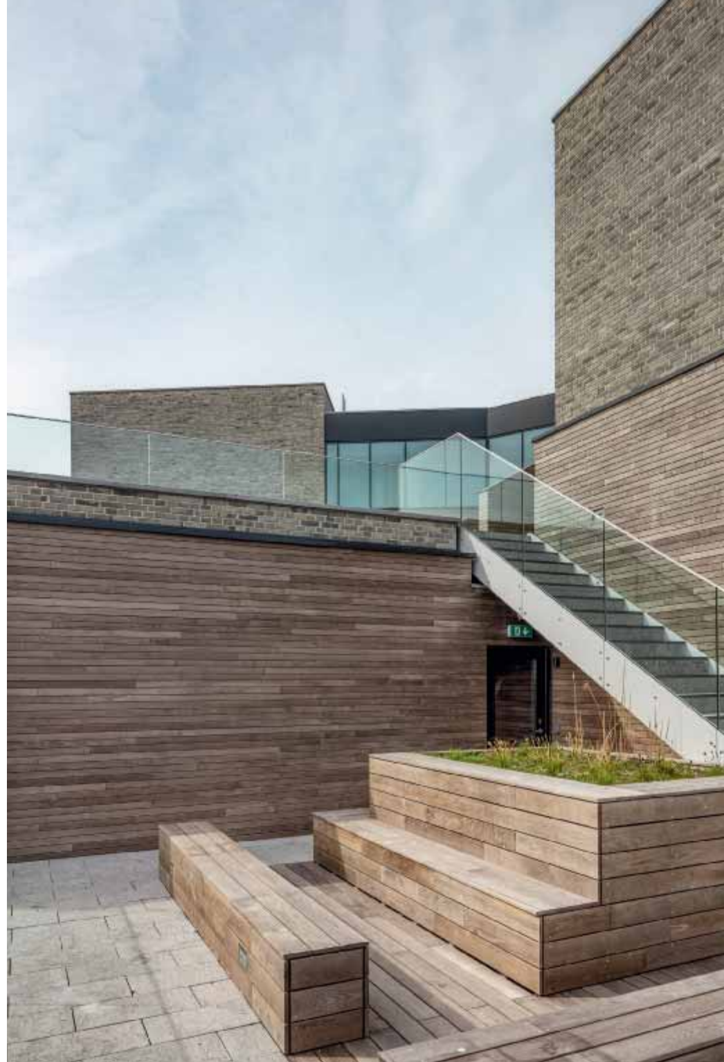
On the top of the building is a large, multi-level communal roof terrace, with plenty of space for relaxation and activities.
