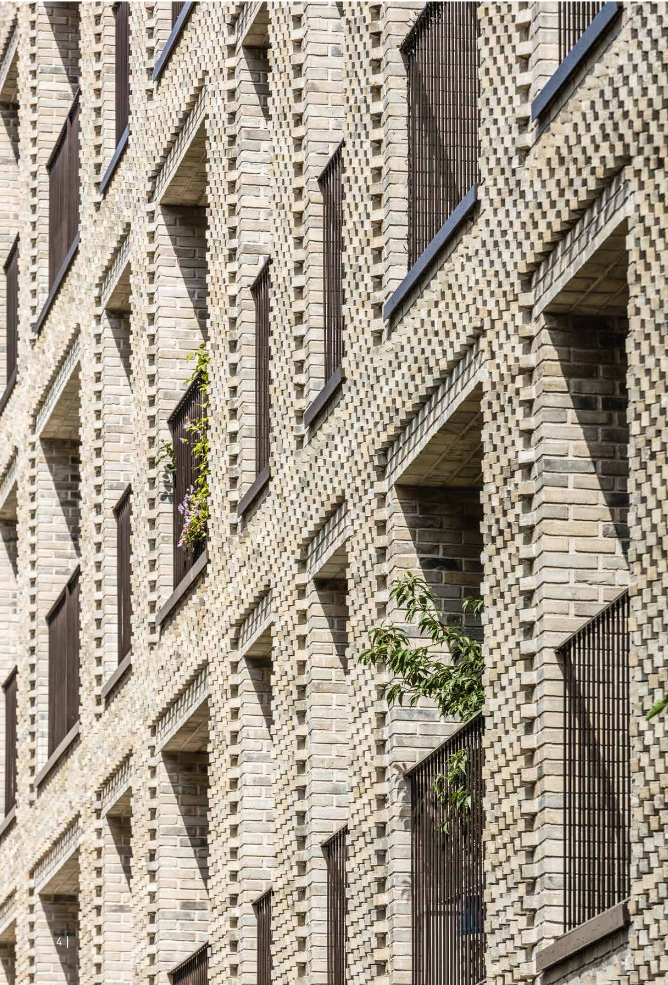
The west façade with inset balconies. The beautiful shadows cast by the brickwork change constantly but are particularly strong in the low afternoon sun.
