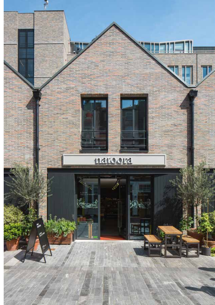
On a number of small houses on Pavilion Road, which runs parallel to Sloane Street, the architects chose a reddish-grey D-brick for the gables.
