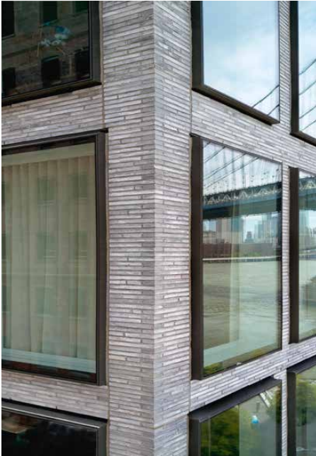
Kolumba has been used in the lower part of the building so that the hand-made brick can be enjoyed from street-level.
