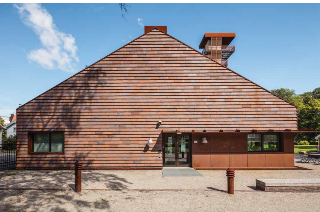
Visitors enter Borgarsyssel Museum from the north. The tight main body of the building has no gutters and a roof pitch of 30 degrees.
