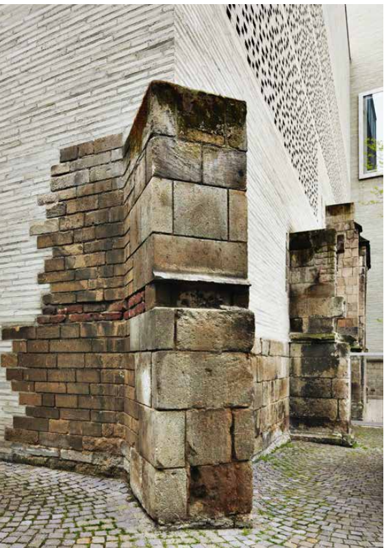
The brick – named after the museum – was ideal because its 40-mm height made it easy to fit in with the ruins' complex and detailed surfaces and shapes.
