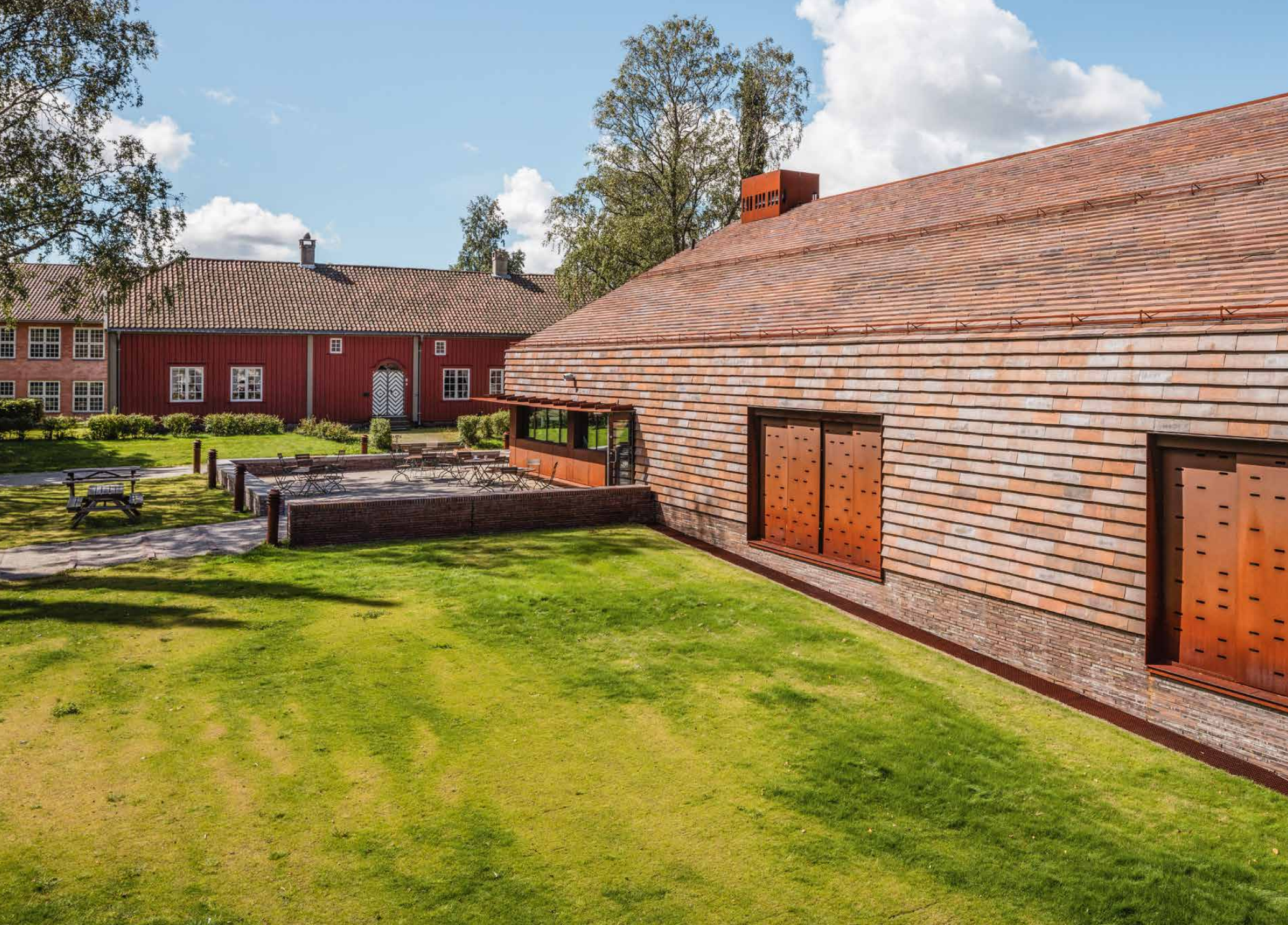
The surrounding terrain falls 1.7 metres from the southeast to the northwest. The slope is occupied by a Kolumba plinth that emerges out of the soil. All of the building elements are made of Corten steel, including the recessed windows, where two rows of perforated shutters can be adjusted to meet the lighting needs of each exhibition.
