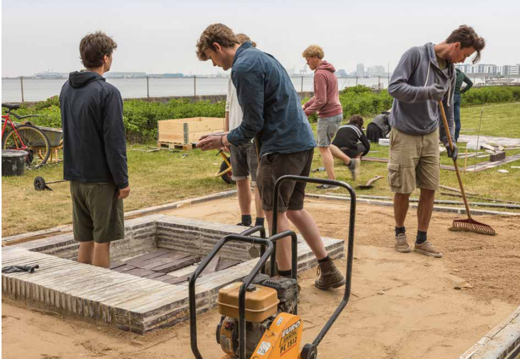
The students had complete responsibility for the job, including laying the bricks for the floor and firepit.
