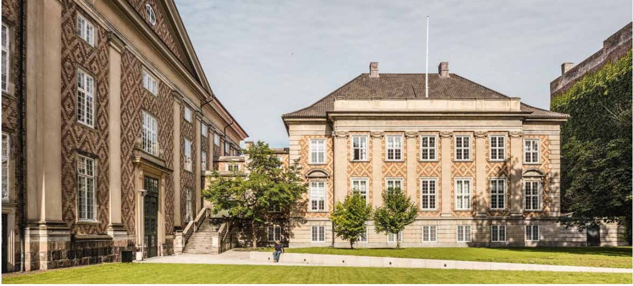
Eastern High Court, Bredgade, Copenhagen. V.L. von Platen, 1702. Extension on the left by Martin Borch, 1903. Photo: Anders Sune Berg.
