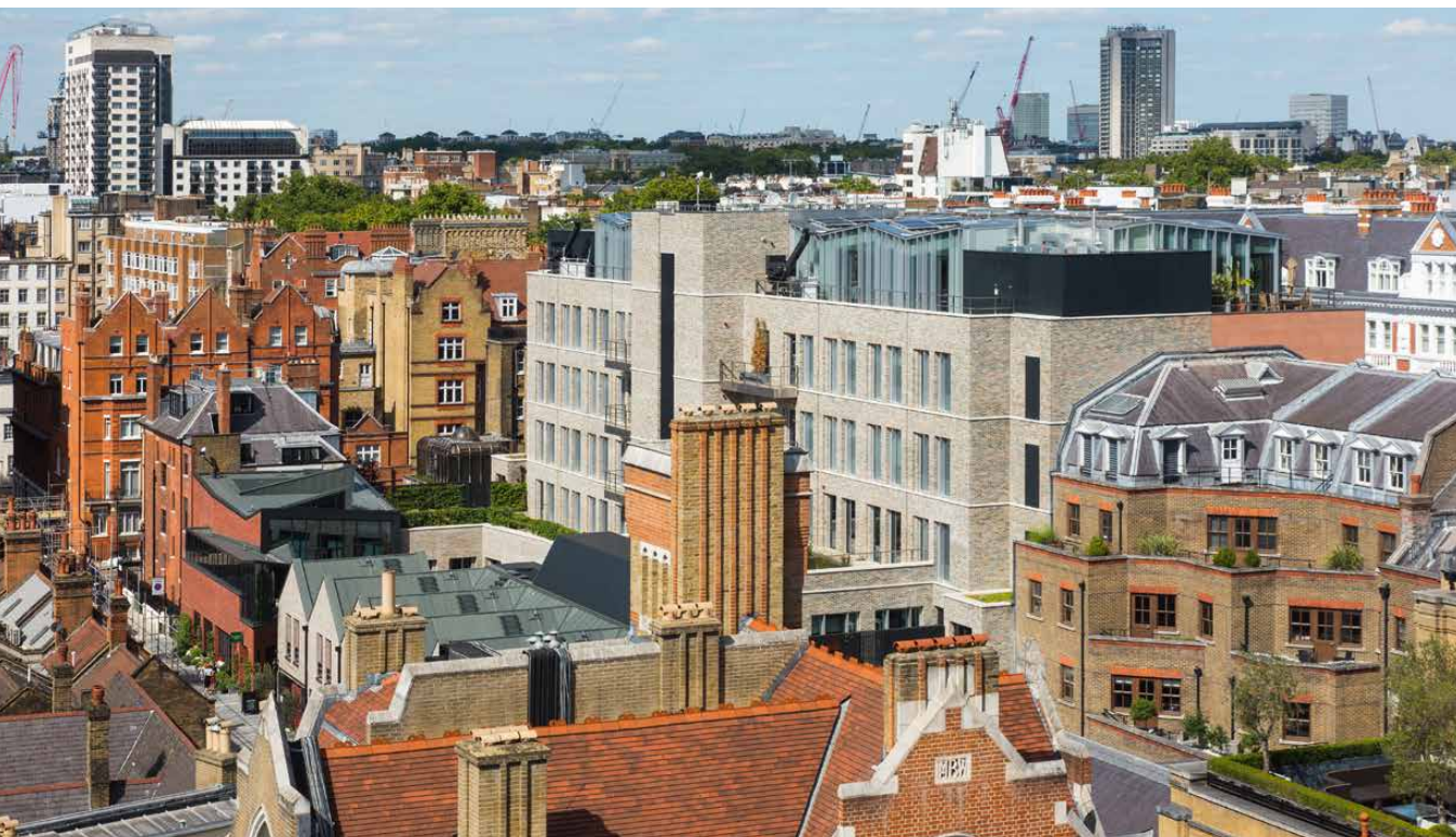
Brick is the dominant building material in Kensington and the obvious choice for most of the new façades.
