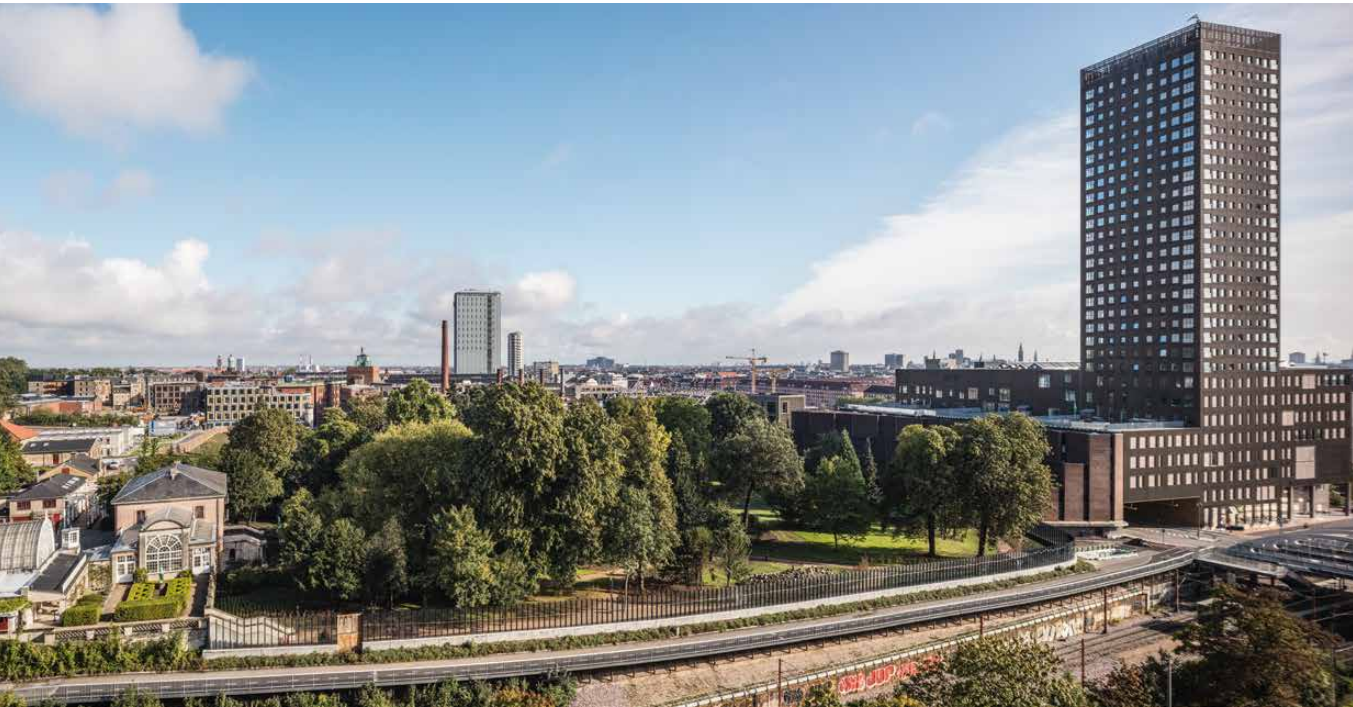
View of the Carlsberg District. On the left, the 1878 home of the founder of the Carlsberg Breweries, J.C. Jacobsen. The garden is now a public park overlooked by the researcher apartments (in the middle of the photo). The 100-metre high Bohr Tower contains apartments and a part of UCC Campus.
