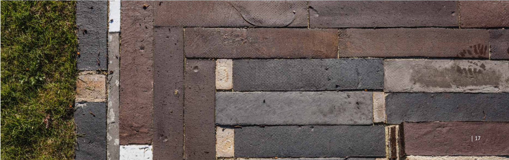
For their firepit, the students chose the hard-fired K57, which can withstand extremely high temperatures. For the floor, they used a combination of K54, D31 and D73 in Flensburg format. The golden and white glazed brick is not only decorative but stands out for people with a visual impairment. The corners are marked with K57 in a herringbone pattern, while the floor is edged with K56 and filled with smaller, glazed bricks – since Kolumba is not modular.
