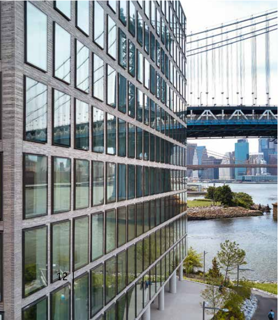
The windows protrude from the façade so that the apartments’ views are unobstructed and not marred by mountings.
