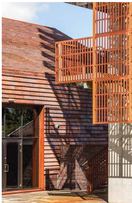
The staircase, which winds its way around the concrete core of the tower is also made of Corten steel.
