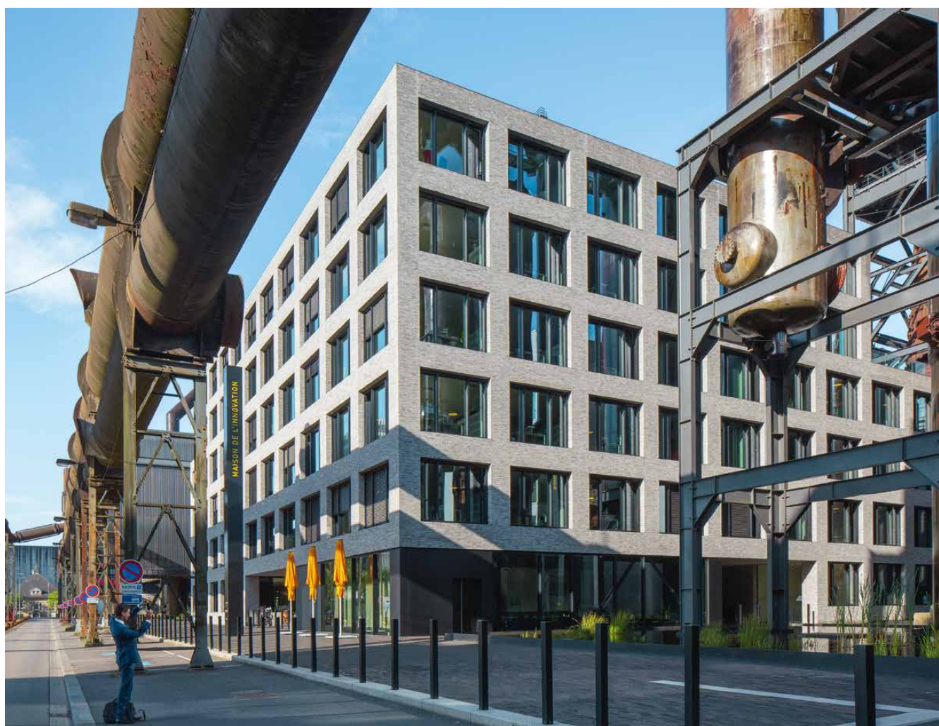
The building volume is clearly defined in order to create a contrast with the crude, preserved parts of the ironworks. The grey brick and mortar façades add to the homogeneity. A wild bond enhances the textual idiom.
