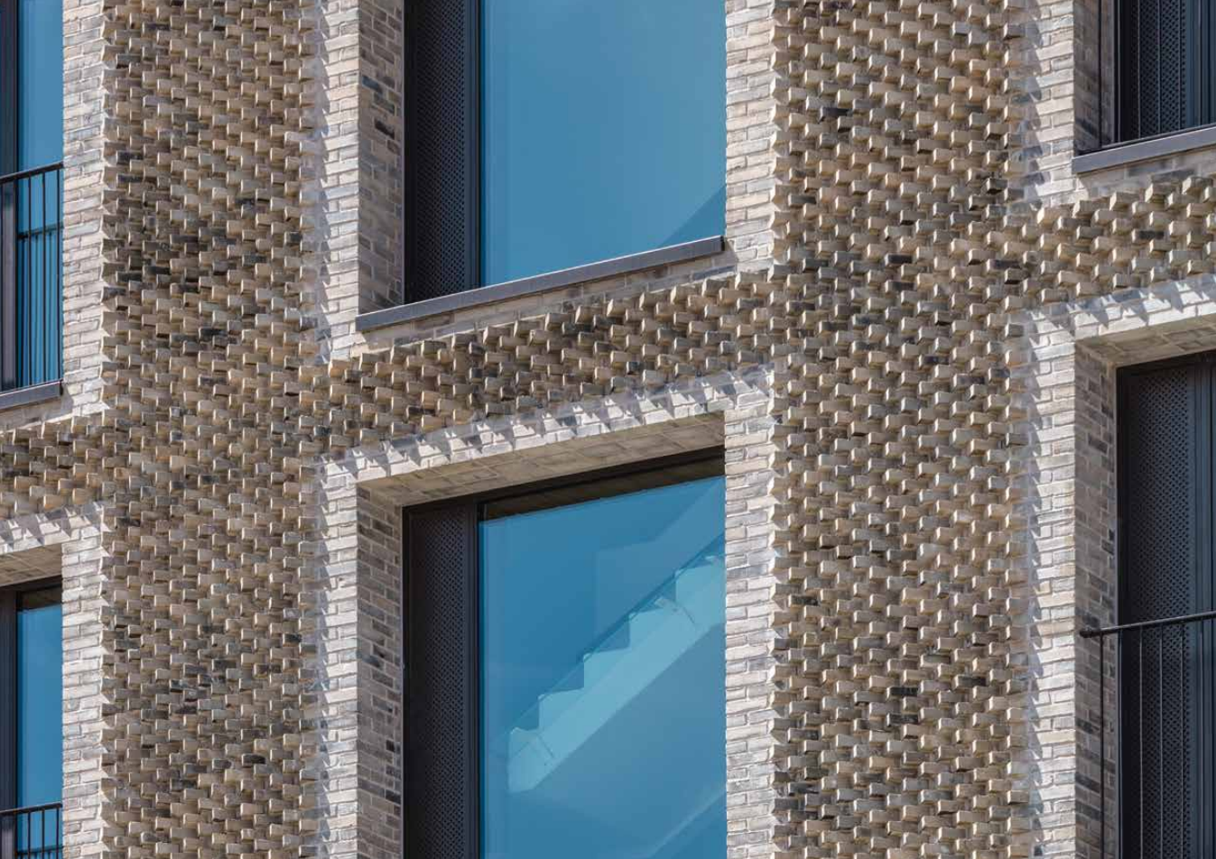
Section of the east façade where the stairs can just be made out behind the window. All joints are recessed, to emphasise the character of the brick.
